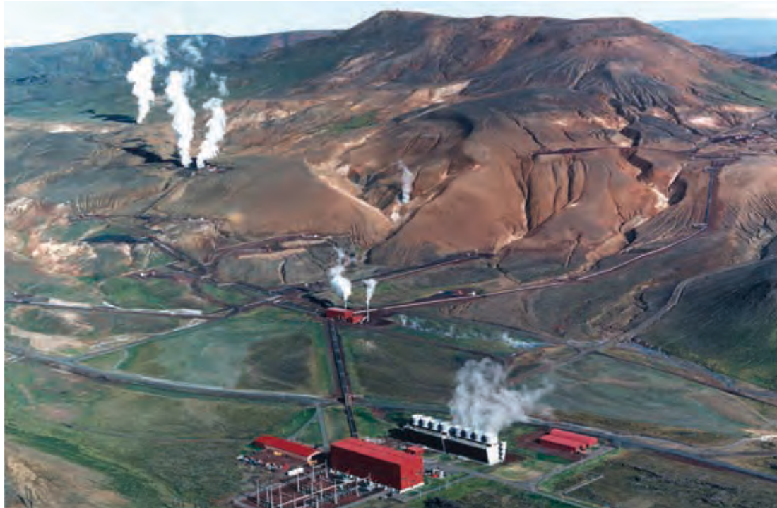
Krafla 60 MW Geothermal Power Plant in Northeast Iceland
